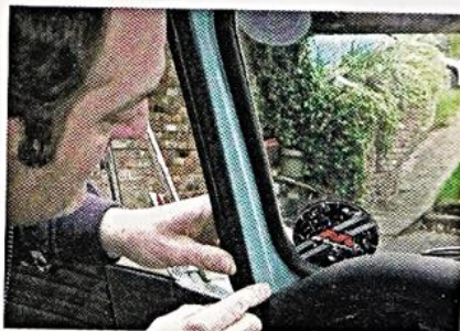
Rot develops where A-pillar meets screen surround inside. It's complicated to put right.
